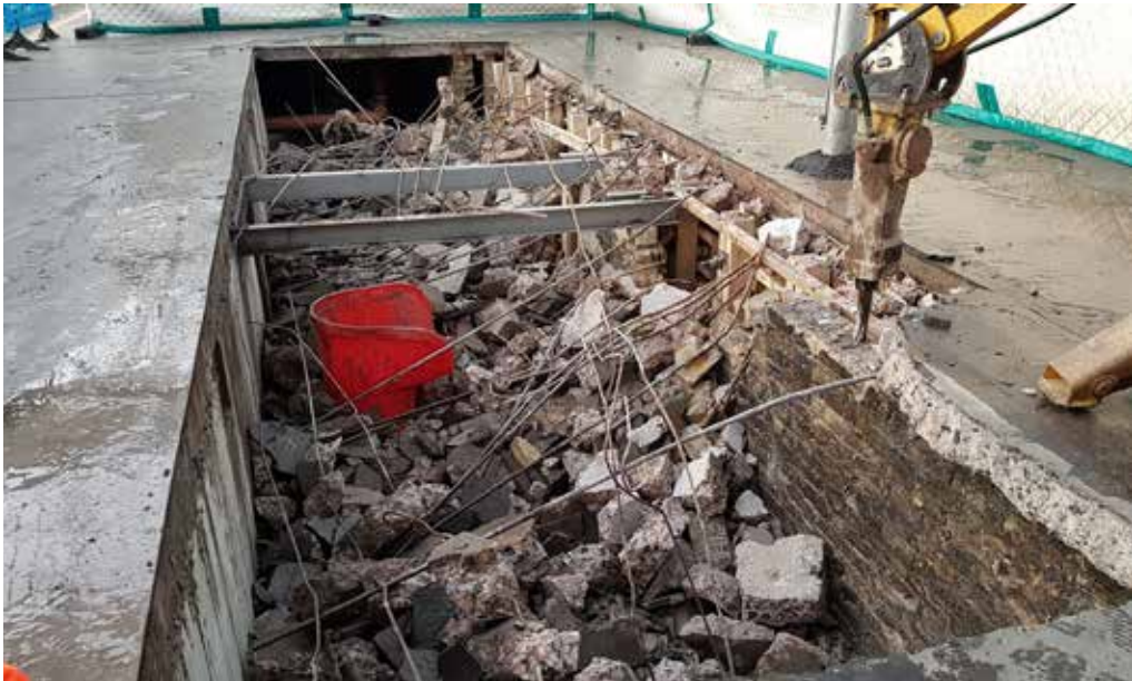
Planning ahead The Waterloo Station concourse slab being demolished to create a new connection to London Underground
