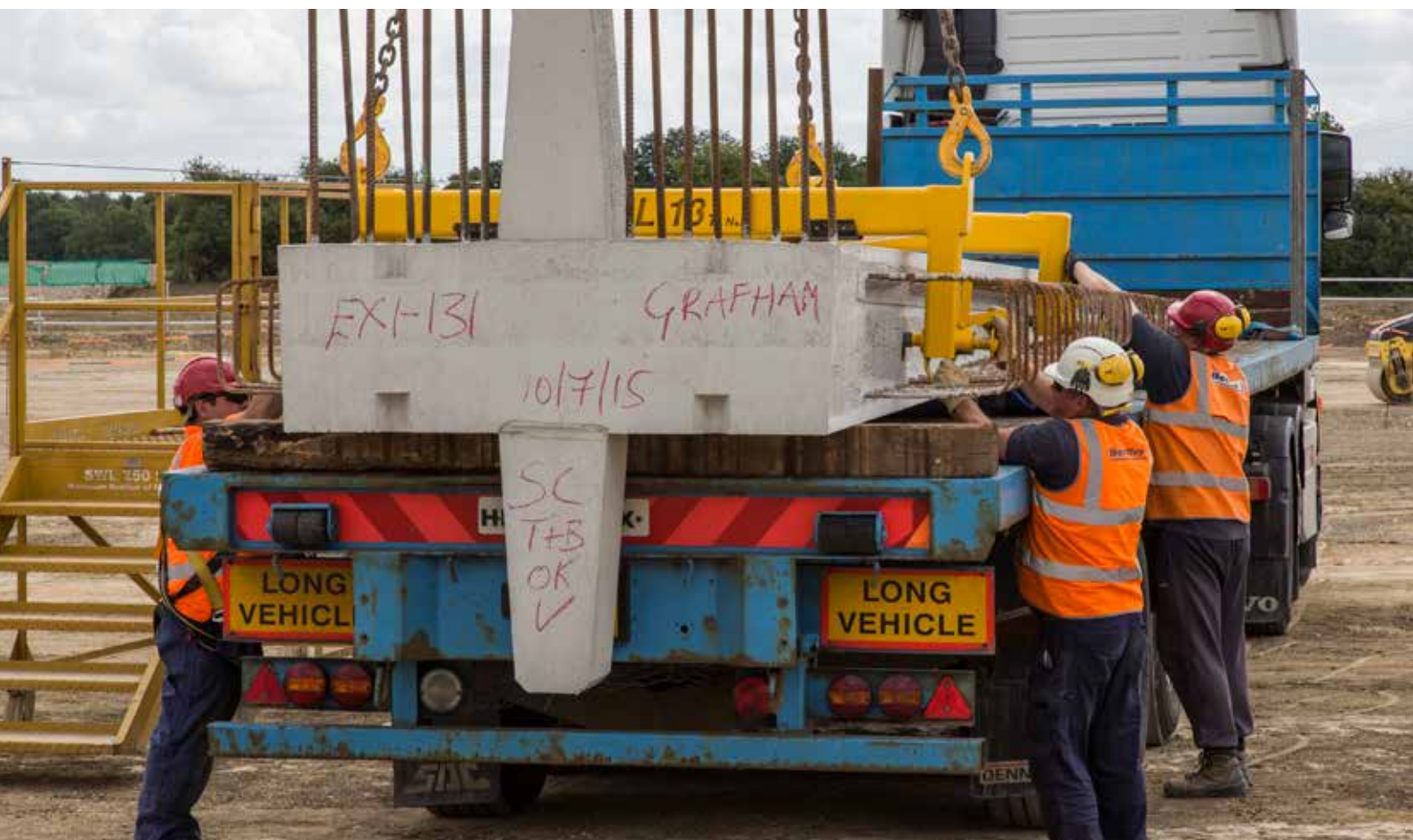
▲ The safe unloading of pre-cast concrete panels at a service reservoir site near Peterborough
