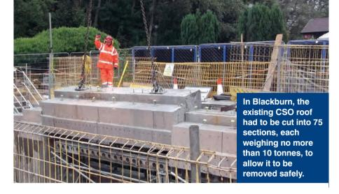
To improve the quality of water being discharged from an existing combined sewer overflow (CSO) chamber, we significantly increased the capacity of the chamber by adding an additional channel, and replaced existing screens. Confronted with a particularly tight site, bound by residential properties, a psychiatric hospital and a river, our team deployed a carefully planned delivery sequence to ensure the works were completed without incident.
