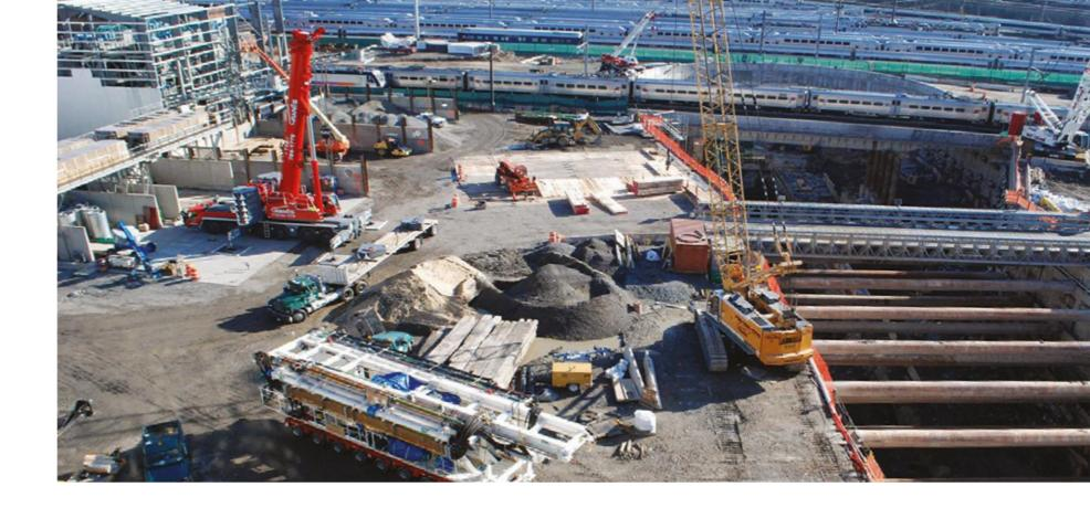
The ESA effectively extends the 63rd Street Tunnel by about 1.6km by excavating new tunnels under the existing bilevel facilities. However, before the project could even begin to tackle these engineering challenges below ground, the junction required extensive upgrades.
