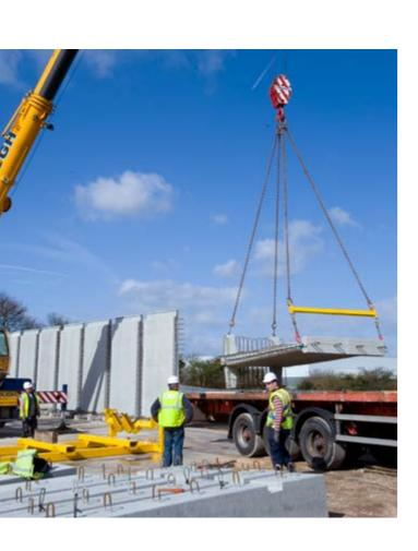
Design for logistics and assembly covers two areas: how a product or system will be assembled and installed, and how it will be transported to site and moved to its intended position as efficiently as possible.
